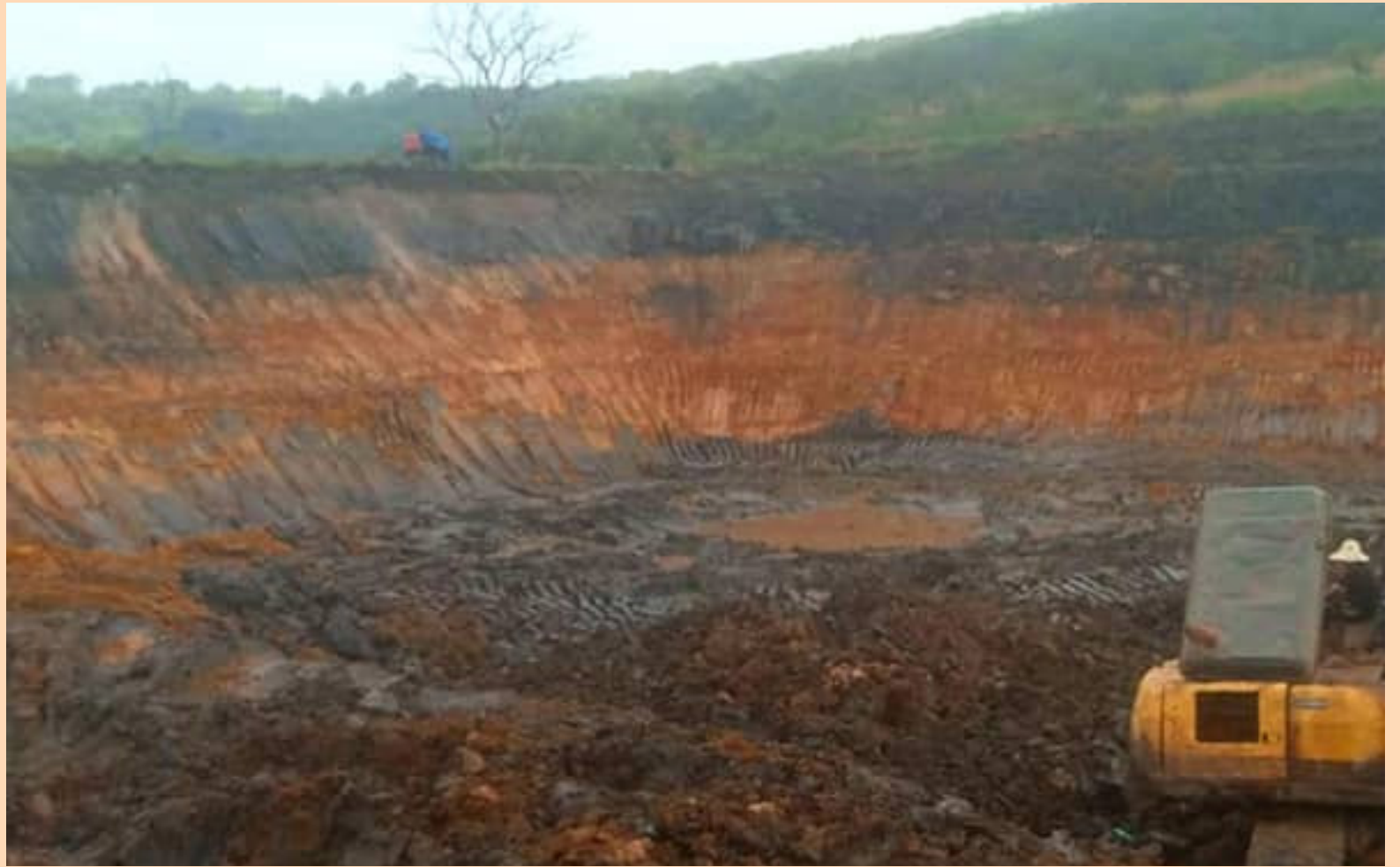
Excavated site on Lake Sonfon
