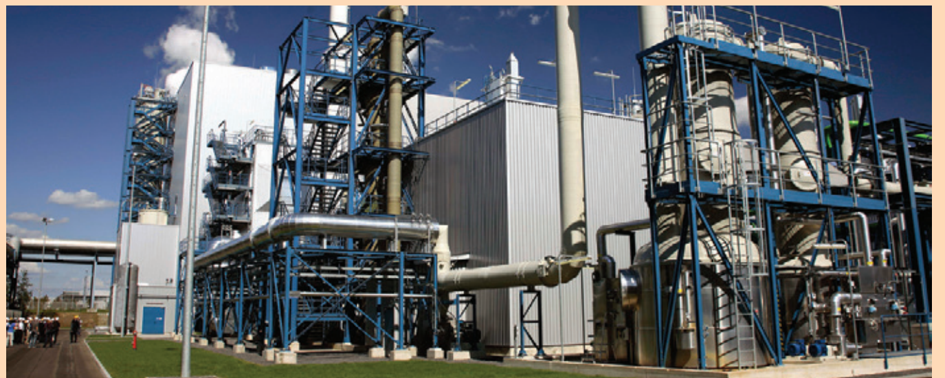
Electric Power Plant
